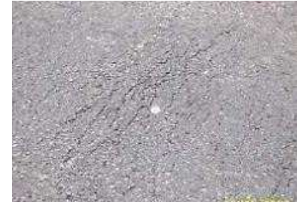
a) Hairline-cracks
