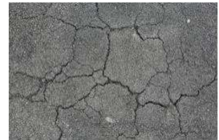
b) Alligator cracks
