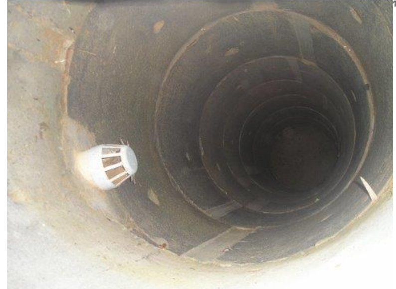
Outlet pipe in recharge well
