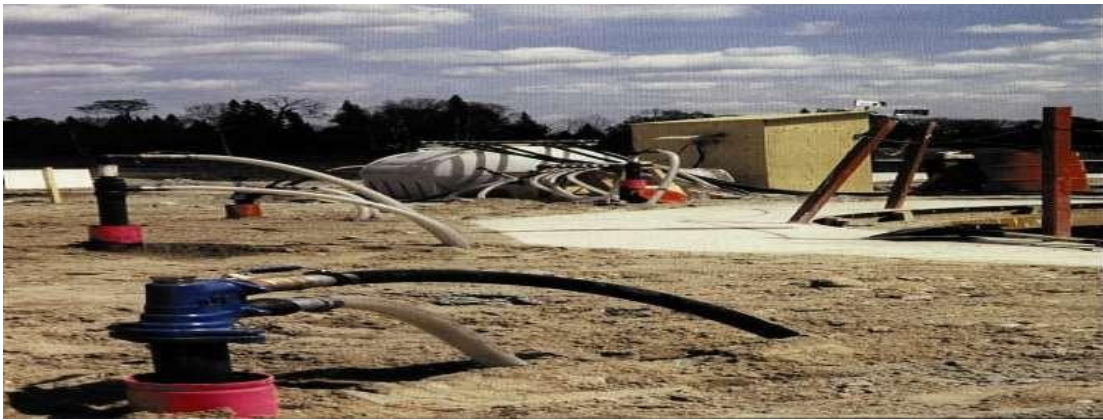
Fig 2.5 Installed Eductor Well Point System
